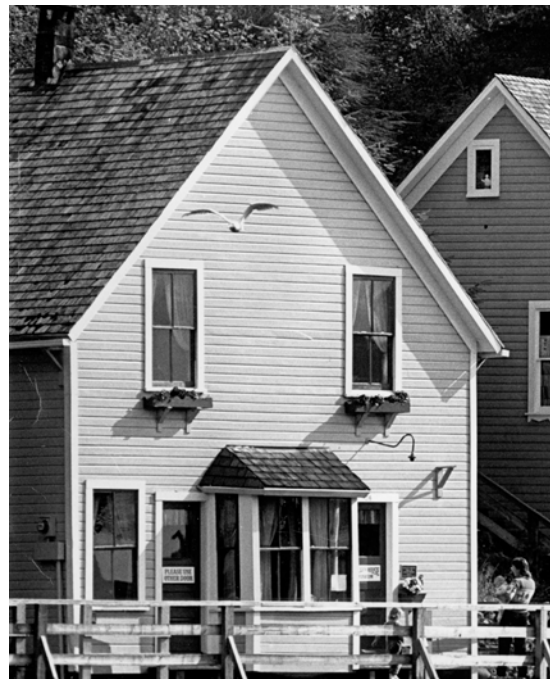
Shortly after restoration in 1976, Dolly's House sports restored siding and window trim and a new cedar shake roof.
