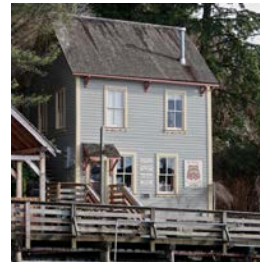
N° 28 Creek Street 1902 This is the oldest remaining building on Creek Street and retains all historic architectural detailing. Pages 24-25
