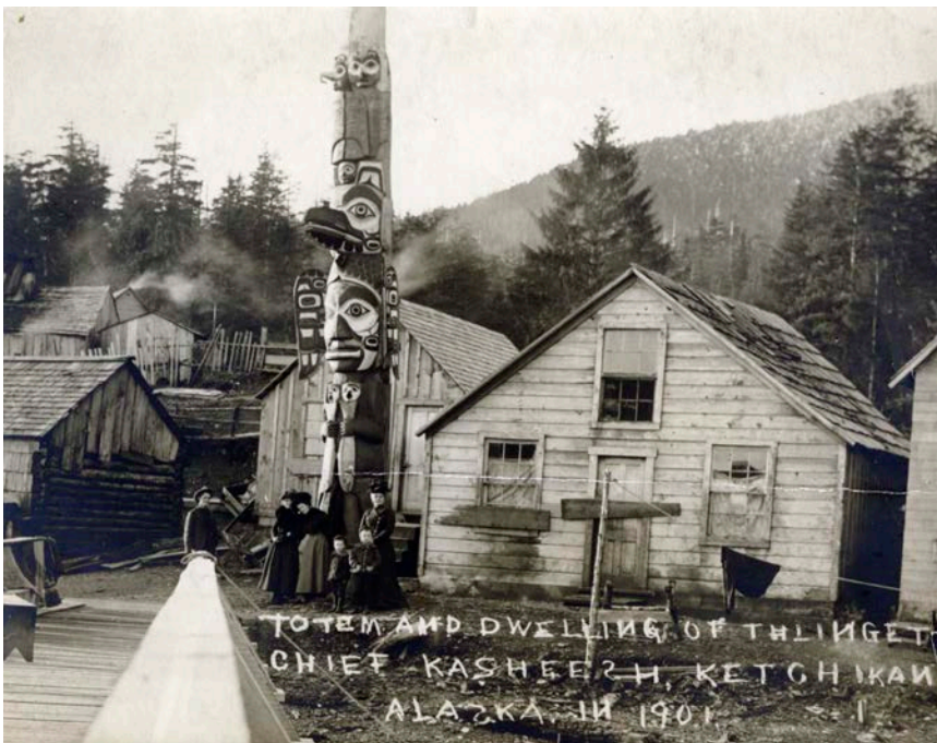
This 1902 village photo illustrates how builders adapted Pioneer style building and milled wood with traditional Native architecture. Early Native houses had doors in the center, flanked by windows on either side, often with another window above the door.
