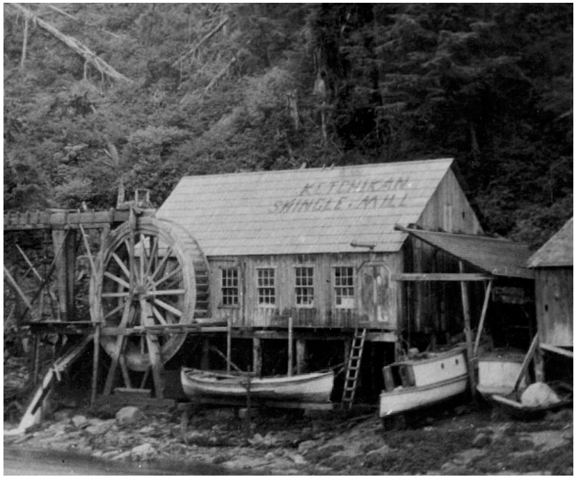
A 700' flume (20" deep and 24" wide) brought water from a point near the present falls to run the water wheel that transmitted power to the mill's saws. The mill building was 24' by 48'. With a crew of 3, the mill produced 10,000 shingles/day.
