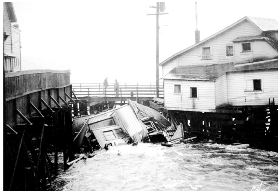
This 1930 photo of storm-swollen Ketchikan Creek documents one of many floods that caused the demise of Creek Street buildings—especially those built on piling over the creek.
