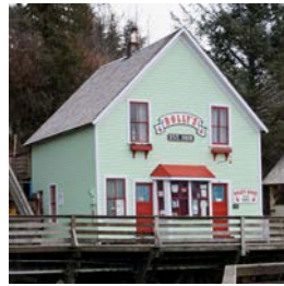
Dolly's House 1905 Dolly's House was the home/business of Creek Street's most famous madame and retains historic authenticity. Pages 22-23
