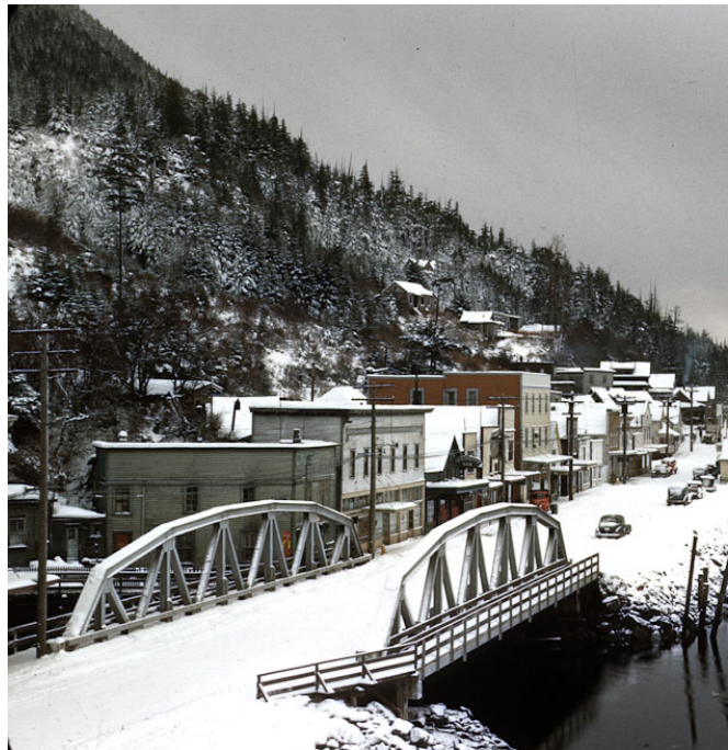
Stedman Street Bridge shortly after construction, circa late 1940s. The wood railing on the walkway was replaced by a steel one in the late 1970s.
