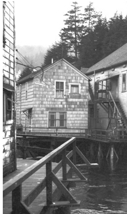
This early 1950s photo shows cedar shake siding then recently installed over the original channel siding.
