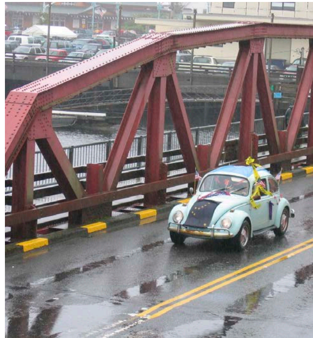
Fourth of July parade, 2006. In 1997, the downstream walkway was expanded to create a popular fishing platform and the bridge was painted its present color.
