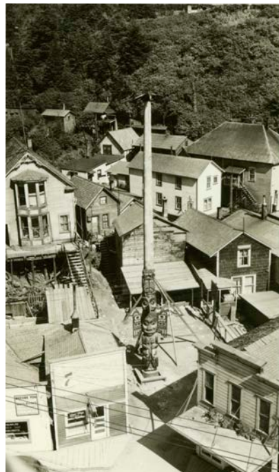
A 1938 view from the new Federal Bldg shows a well-maintained N° 4 and dense buildings on both sides of the Creek.
